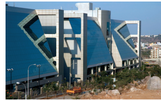
Figure 11.43 The Cyber Gateway Building in Hyderabad's Hitec City. The complex houses firms like the multinational software companies Microsoft, IBM, and Toshiba, as well as Indian companies like Wipro, which provides information technology services and product design. Hitec City also houses professional schools in business and information technology.
