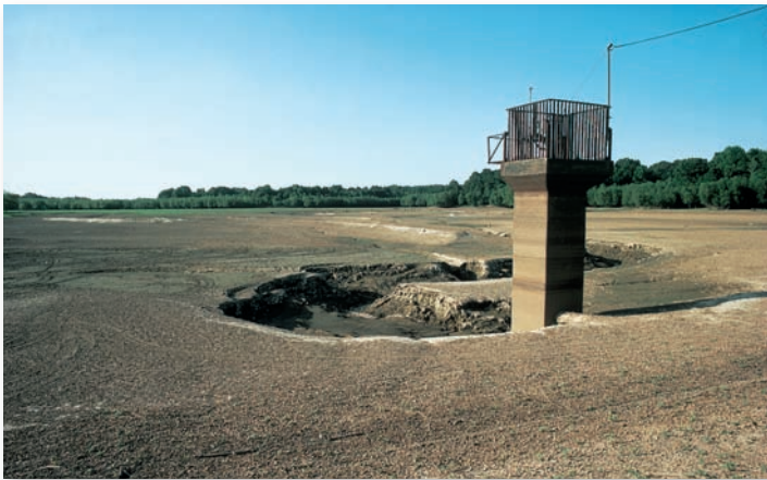
FIGURE 17.21 This dam is now useless because its reservoir has filled with silt and sediment.
