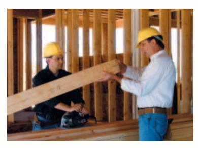
↑ Check stock before cutting it. Nails, cracks, or loose knots could cause a power saw to kick back or send pieces flying out at high speed. Before starting to cut, put on safety goggles.
