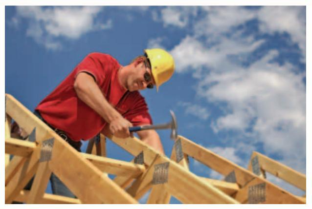
★ This carpenter is nailing roof trusses. Why should eye protection be worn when using a hammer?
